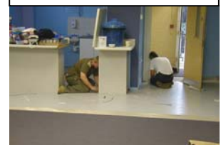
The new floor is laid
